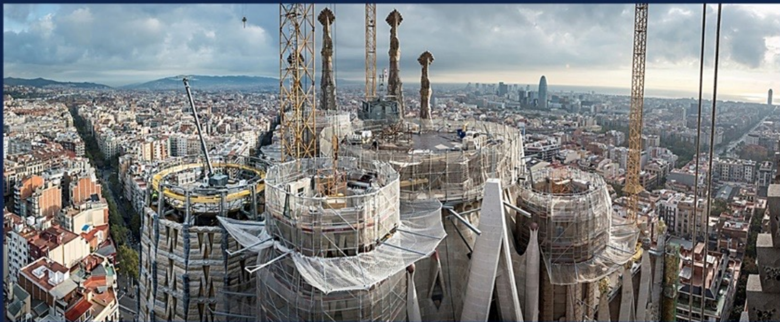
Tower Modular Construction
