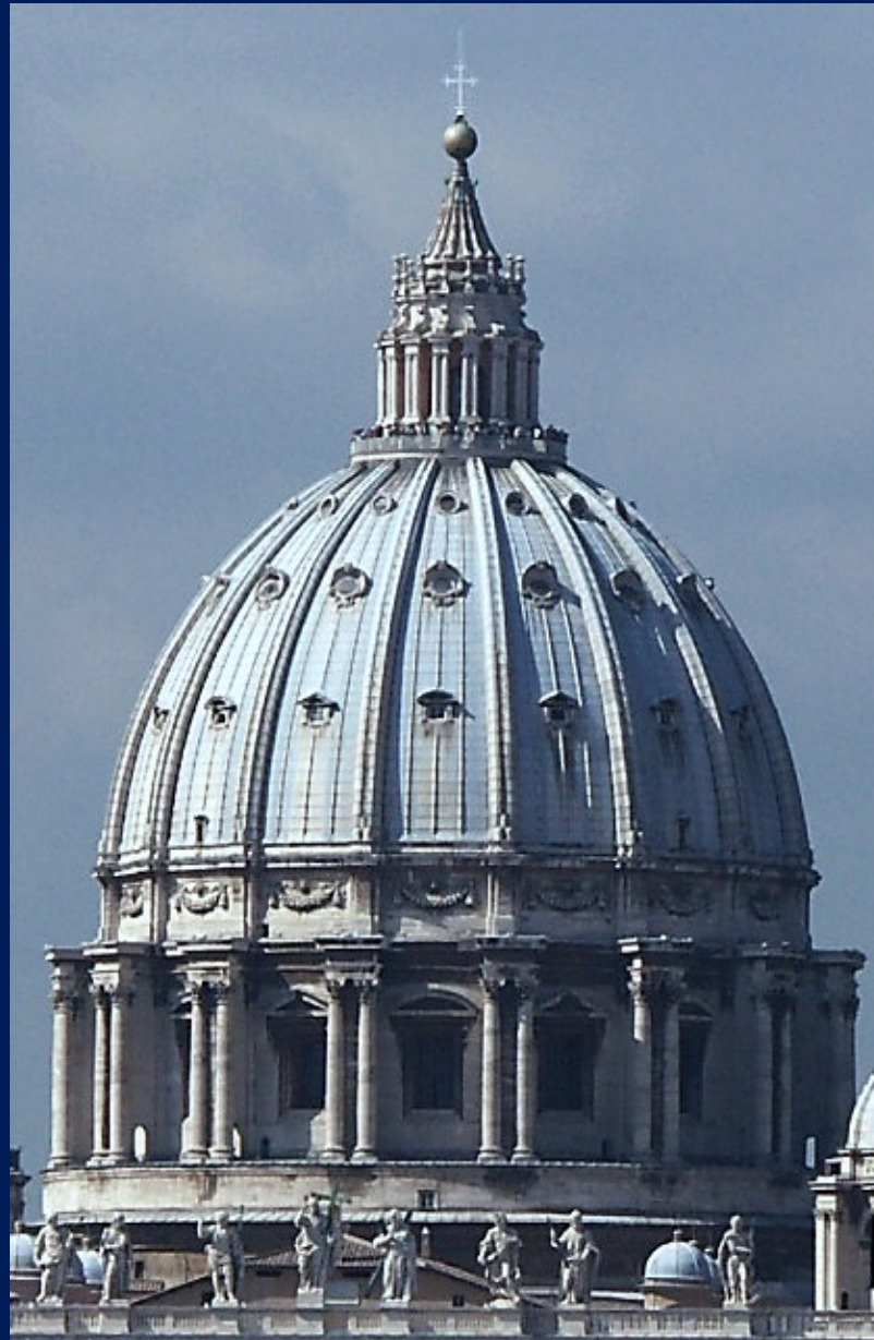
Dome of St. Peter's Basilica
