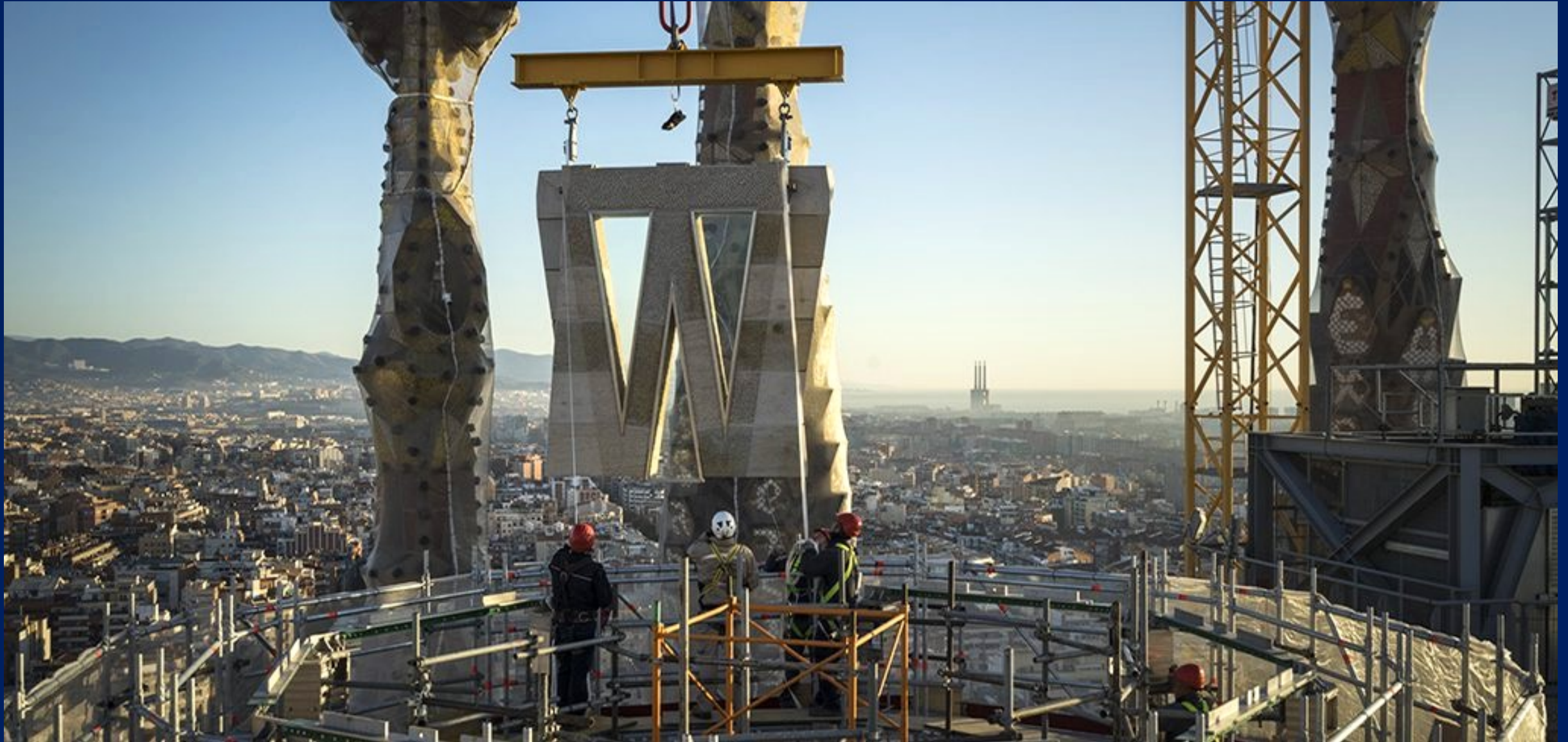
24 tons lifting – French Mother-crane stands at 180m height, handles 1mm tolerance for fitting prefabricated units.
