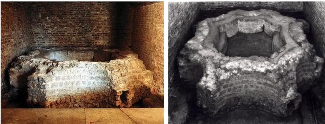
In the foundation section of the baptismal pool there is below to the right a drainage outlet. On the exterior there is a rectangular opening which is visible on the inside with a lead pipe; this was connected to a channel which is now lost. The supply of baptismal water might have come from a stream above the basin edge located in the back to the left. (SR)
